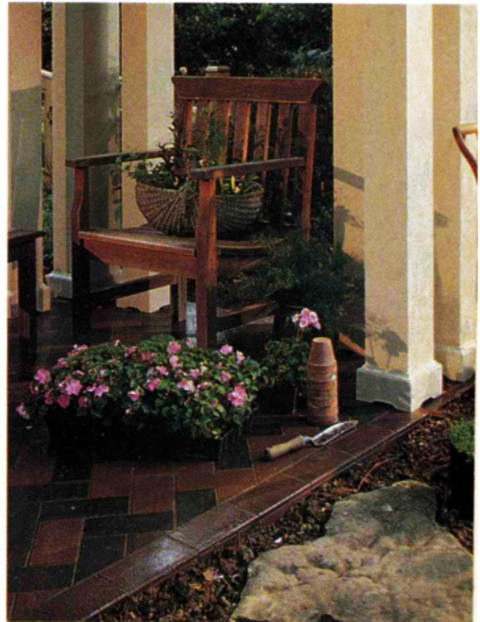
Brick coping dresses up the edge of the flooring and helps hide the concrete slab underneath.
